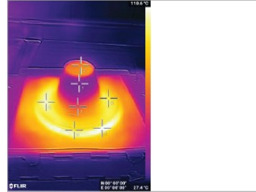
Latitude: N 00° 00' 00", Longitude: E 00° 00' 00" flir_20221106T173413.jpg
