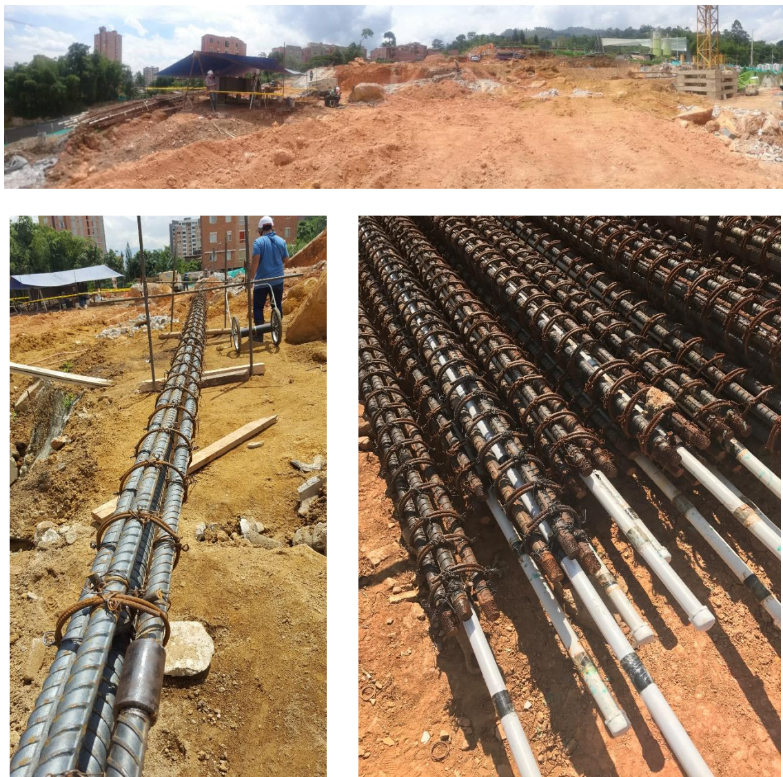
Fig. 15. Site conditions and micropile's reinforcement.
