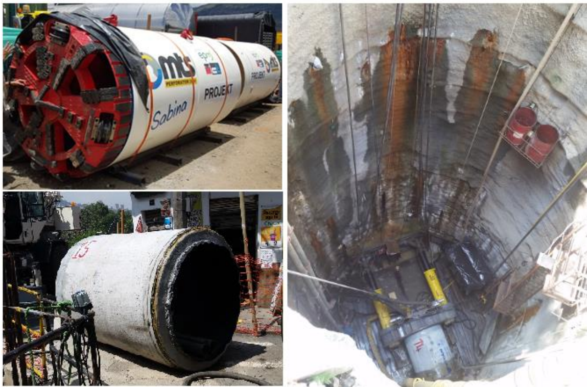
Figure 20. Launch shaft, concrete pipes and hydraulic jacks used in “Centro Parrilla” Project. Modified
