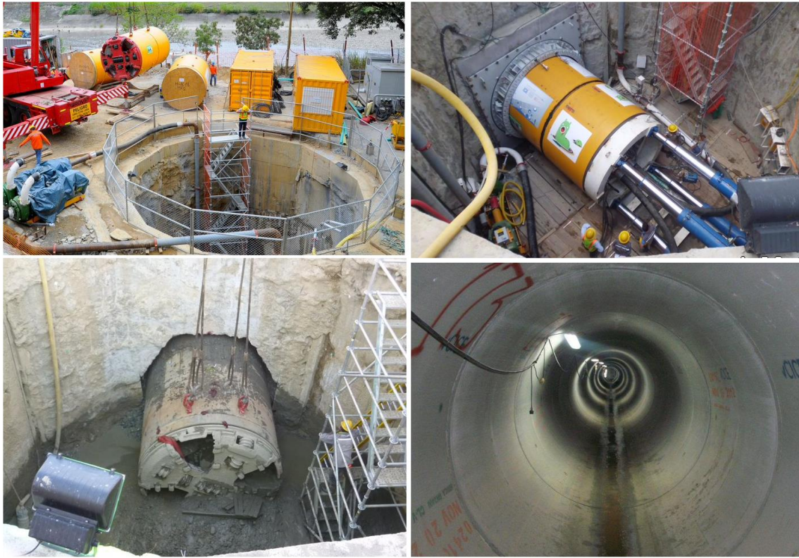
Figure 29. Typical shaft, TBM, hydraulic jacks and concrete pipe used in the “Interceptor Norte” project
